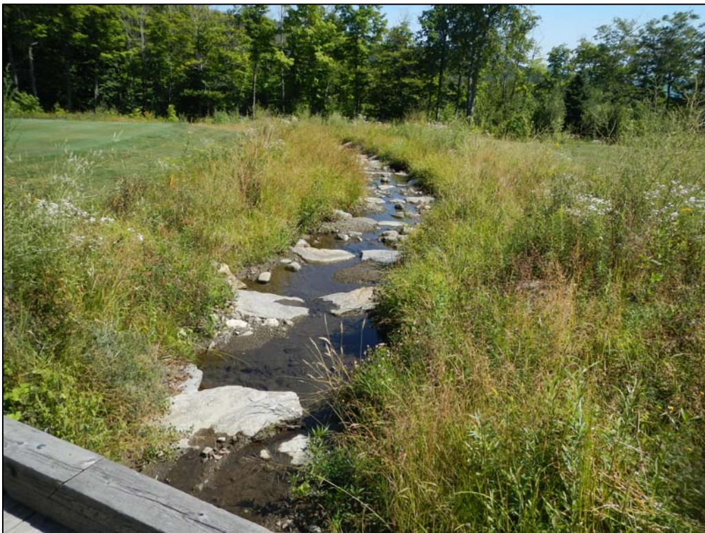
Photograph 18: P2-TB1 looking downstream from Station P2-TB1-P1, facing northeast (C. Martin, 8/8/12)
