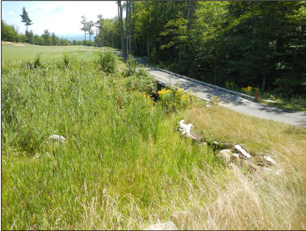
Photograph 11: H4-WT1/2 from Station H4-WT1-P1, facing southeast (C. Martin, 8/8/12)
