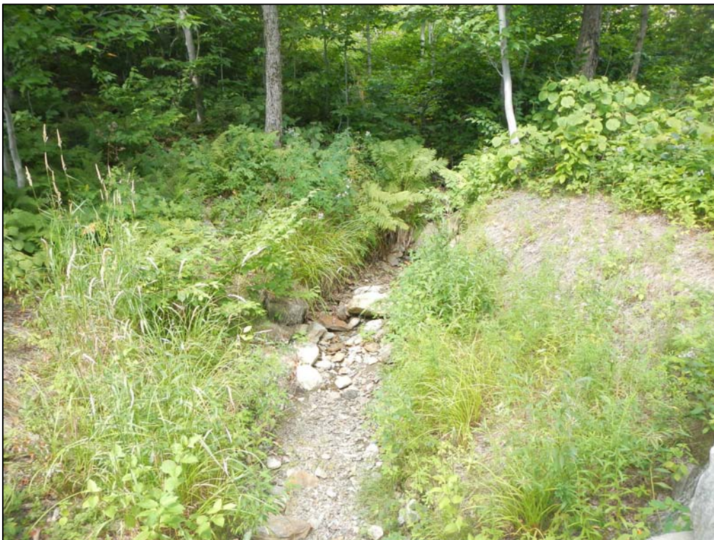
Photograph 40: H13-TB1d from Station H15-TB1d-P1, facing north (P. Werts, 8/8/12)
