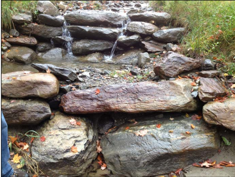
Photograph 3: P2-TB1, Upstream of cart path, front of two grade-control structures with excess material to be removed (PBW, 10/4/12)
