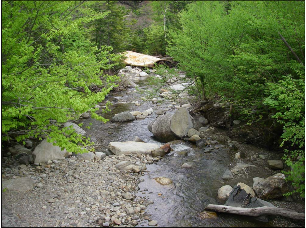
Photograph 9: Former culvert under cart path near Hole 10, blown out by Tropical Storm Irene, remains in channel (PBW, 5/23/12)
