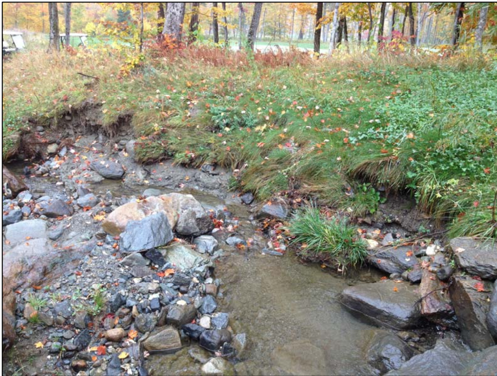
Photograph 2: P2-TB1, Upstream of cart path, two smaller areas of erosion (PBW, 10/4/12)
