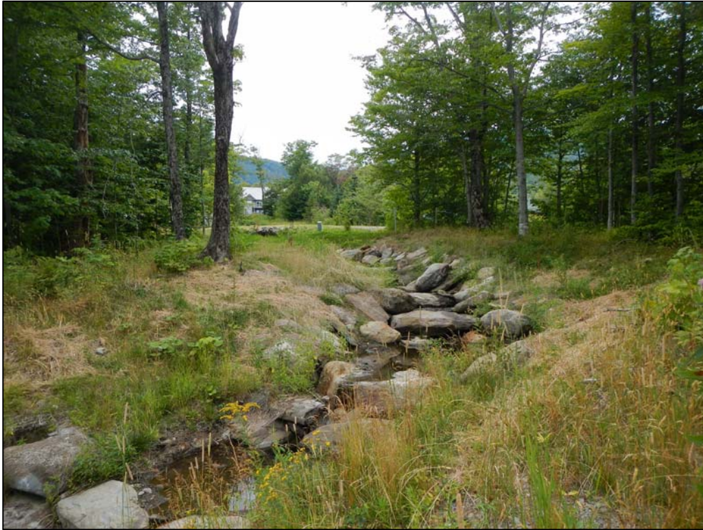
Photograph 19: P2-TB1 looking upstream from Station P2-TB1-P2, facing southwest (P. Werts, 8/8/12)
