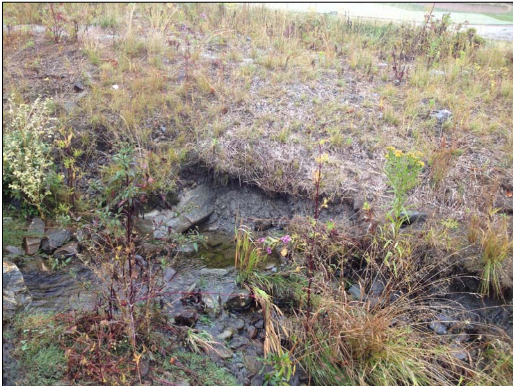
Photograph 8: H16-SC1, small area of erosion (PBW, 10/4/12)
