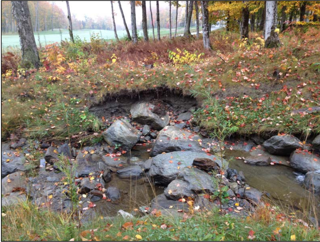
Photograph 1: P2-TB1 Upstream of cart path, main area of erosion (PBW, 10/4/12)
