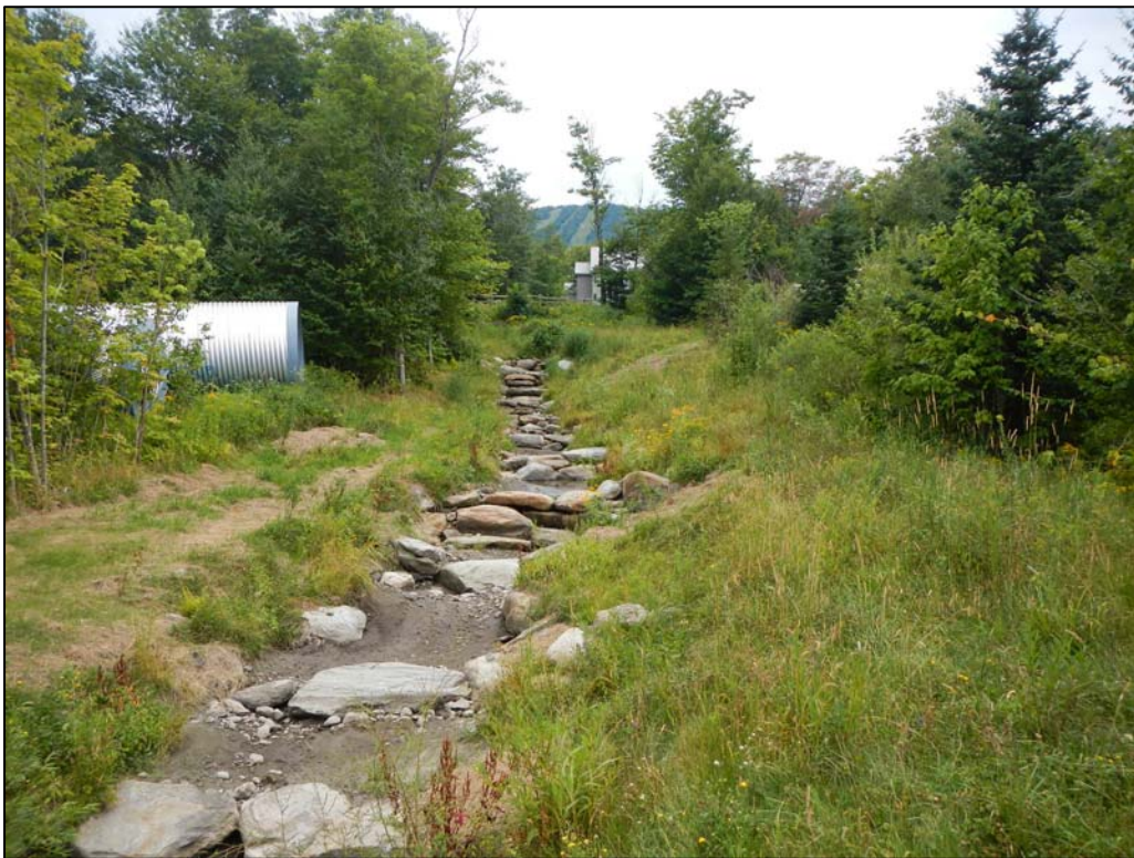
Photograph 20: P2-TB1 looking upstream from Station P2-TB1-P3, facing southwest (P. Werts, 8/8/12)
